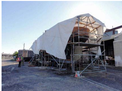
Julie Burgess Project underway in Devonport
