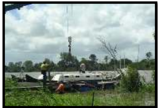
Launching with a Crane – That's a first!
