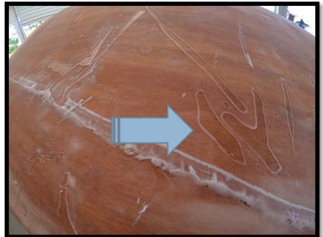
The result is divots that will have to be filled and sanded
